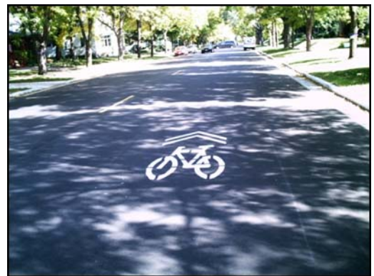
Example of a bike “sharrow” indicating a shared roadway
