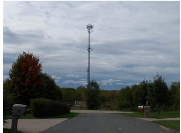
Communication Tower in T. Greenfield
