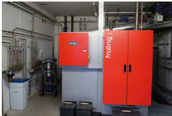
Figure 29 – Froling TX 150 Pellet/Chip Boiler
