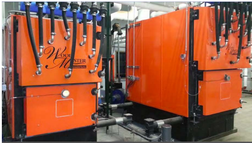
Figure 40 – Wood Master Boilers
