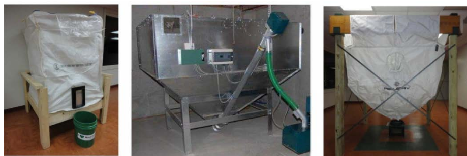
Figure 25 – Bulk Pellet Fuel Delivery & Storage Units
