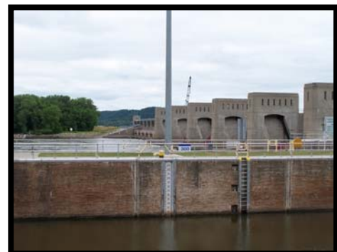
Mississippi River Lock and Dam 9
