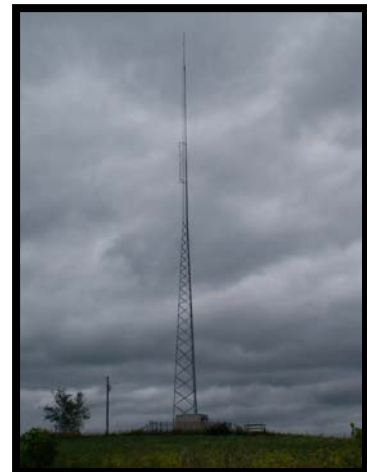
A cell tower in southern Crawford County
