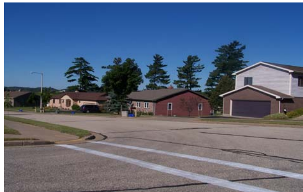
Department of Defense Sponsored Housing Project in Tomah
