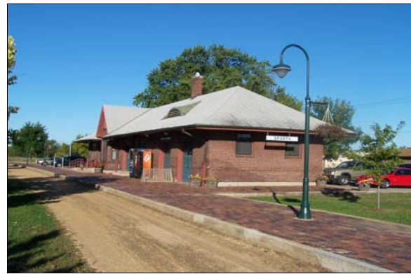
Remodeled Depot serving as a rest stop and information center on the famous Elroy-Sparta bike trail
